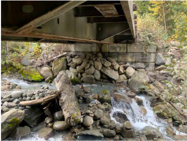
Left Bank Abutment when facing downstream
