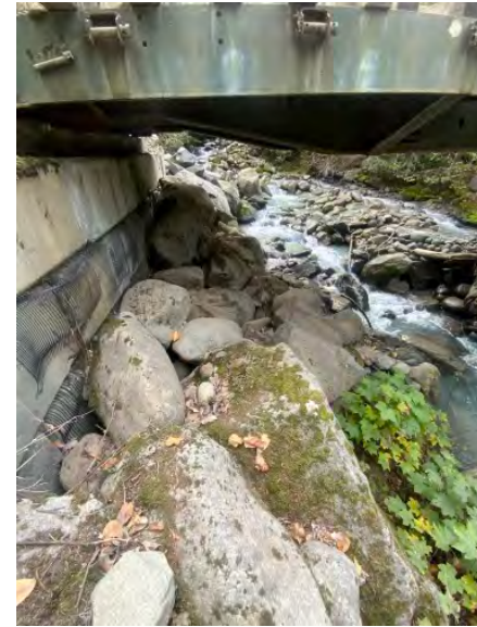
Right Bank Abutment when facing downstream
